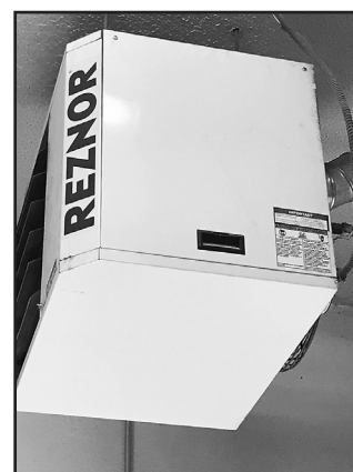
Reznor Garage Heaters (5)
