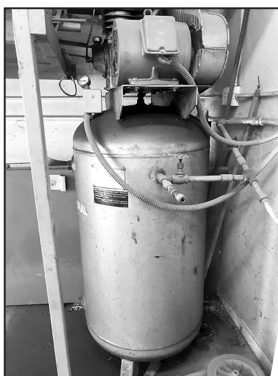
Large Commercial Air Compressor
