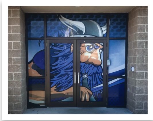
Window wraps at both Northwood-Kensett school buildings support campus security efforts
